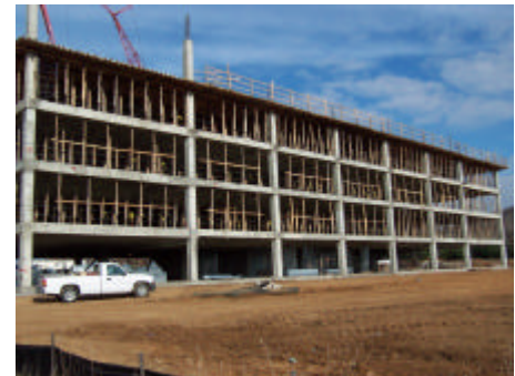
Highwoods Cool Springs III Construction Inspection and Geotechnical Engineering
