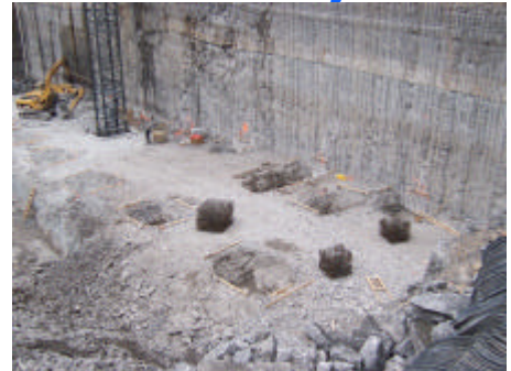
Suntrust Plaza Geotechnical Engineering
